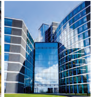
HELISFYR ATRIUM, OSLO, NORWAY
